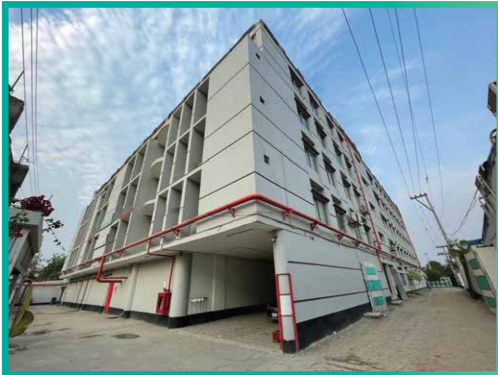
Factory: M H Tower, 21 Vogra, Gazipur sadar, Gazipur
